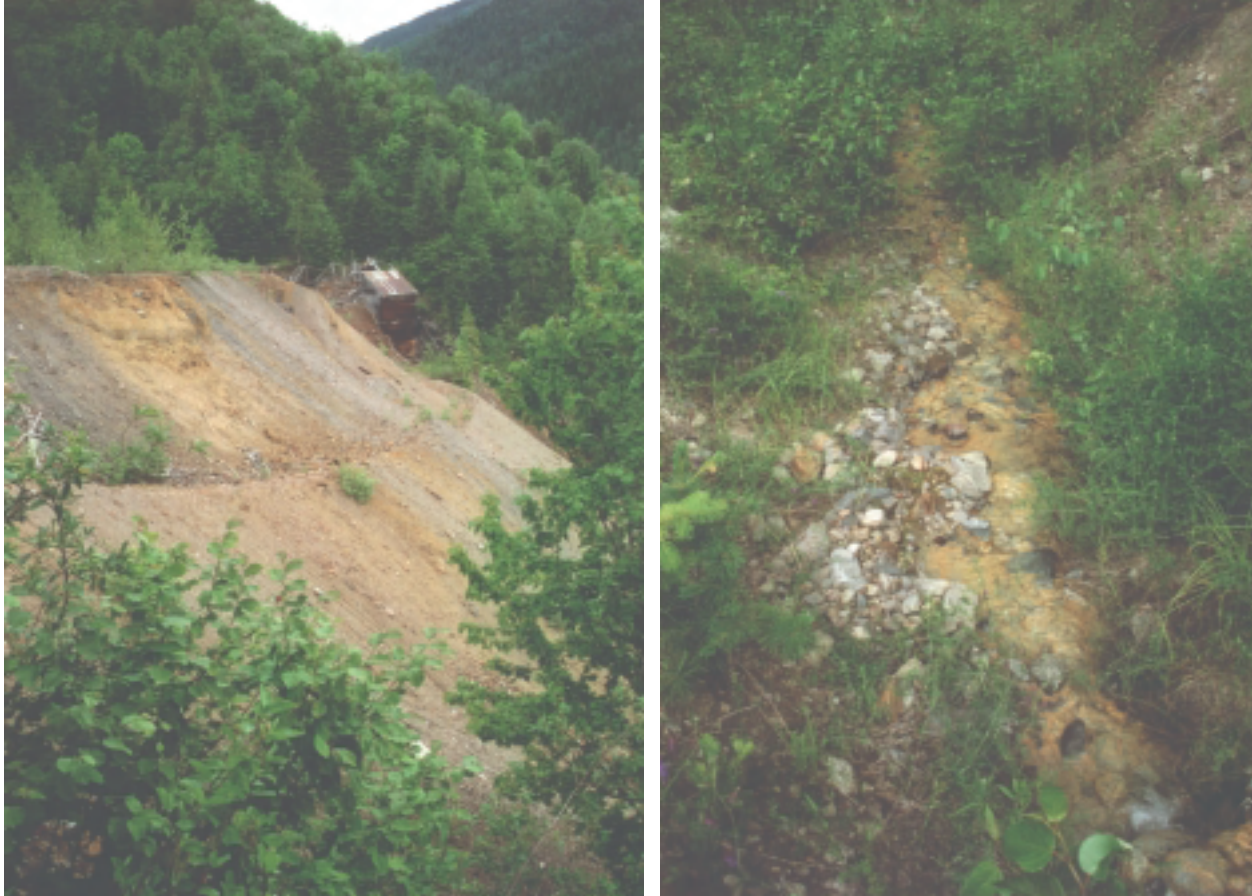
Waste dumps and runoff on Mt. Dundee
