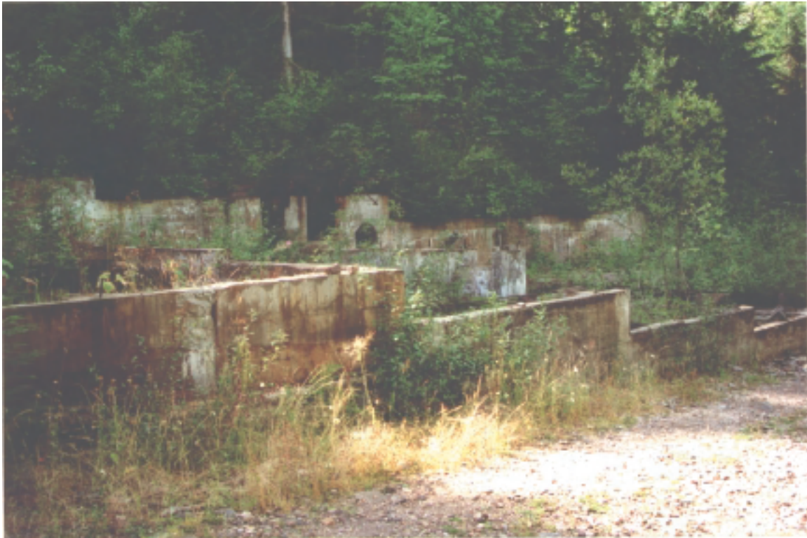
Foundation of historic Queen Mill
